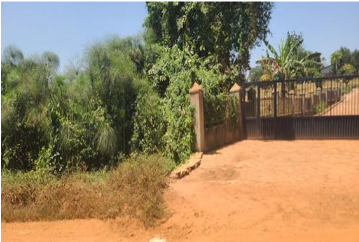
Plate 2: House constructed in a wetland
